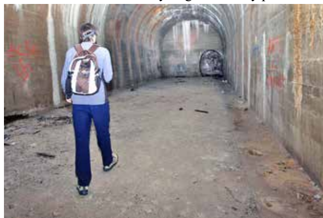
Looking north along last concrete-lined chamber in Bunker 1. Beyond this a narrow unlined tunnel leads to an unfinished stairway to the surface. Photo Žiga Ribič
